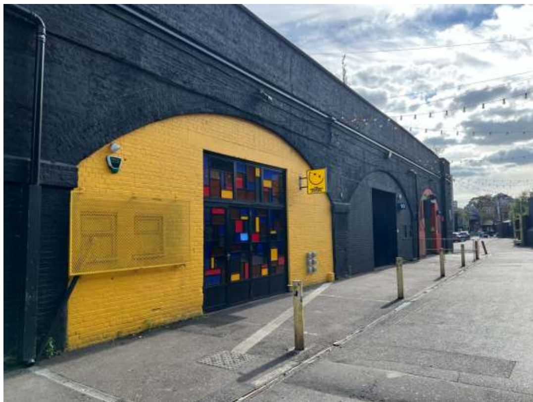
Figure 1: Arch 11 on Bohemia Place
